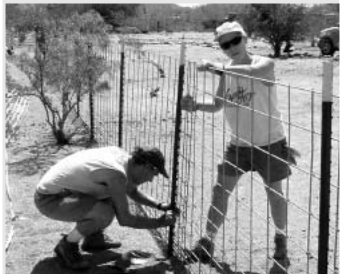
Mike & Jean at the Annex Working on the New Perimeter Fence
